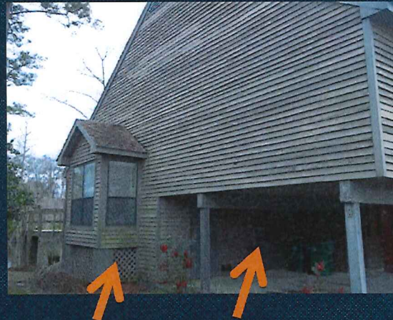
Crawlspace and Enclosure
